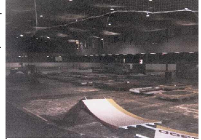
Sports Plus roller hockey rink under construction
